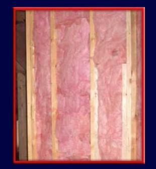
• The insulation is packed into a building's outer walls and attic, where it reduces the flow of heat between the building and the surrounding air.
